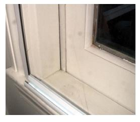
My first window was a hybrid: Windowsavers magnetic strip for the sides and top, and a Modern Plastics extrusion for the bottom, which fits flat on top of a window sill (See diagram 1.) Works well, looks good, but somewhat expensive and time-consuming to build.
